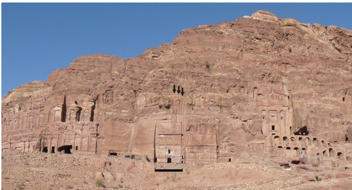
Figure 1. The Royal Tombs assemblage where the Silk Tomb (marked in the figure) is located. An area of intense breakdown of drainage channel is also marked.
