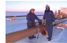
Photo Courtesy of Tylon International Radiography of weld joints.
