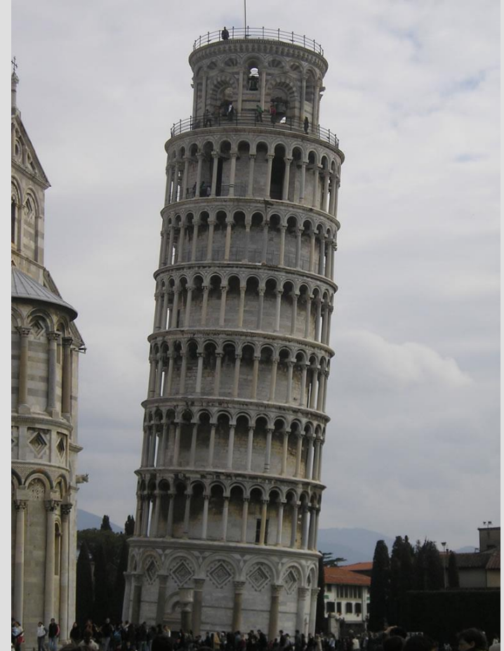
Leaning Tower of Pisa
